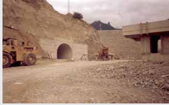
Atasu Barajı Dipsavak Tüneli Trabzon/TÜRKİYE Atasu Dam Bottom Outlet Tunnel Trabzon/TURKEY
