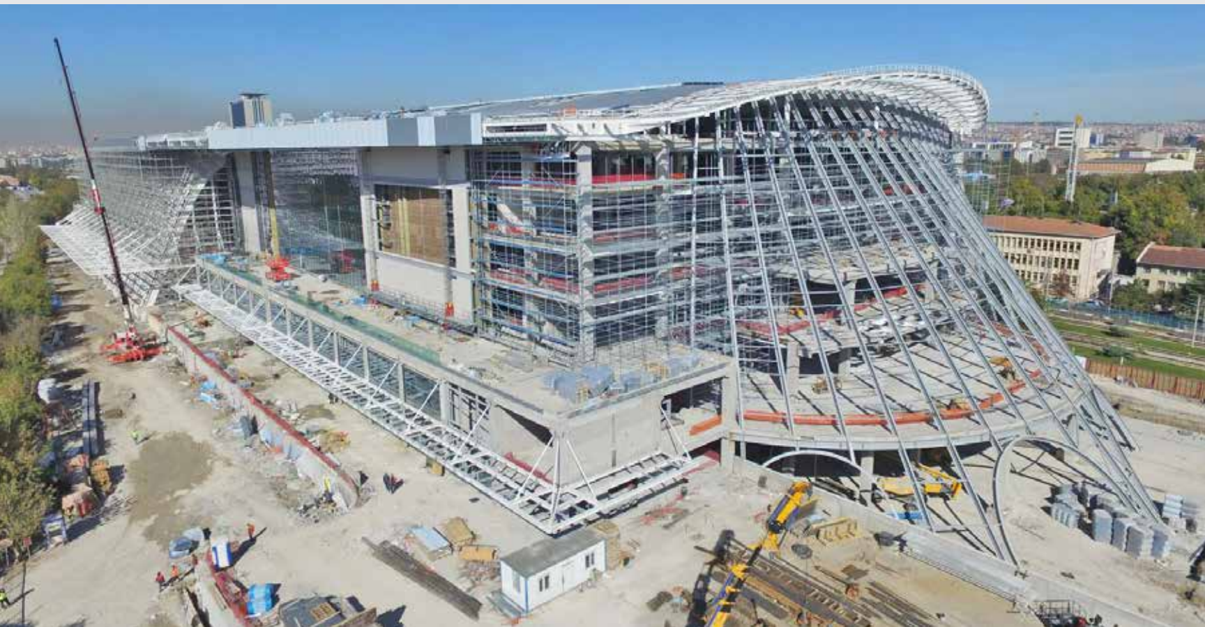
Ankara Hızlı Tren Garı Çelik İmalat ve Montajı Ankara/TÜRKİYE Ankara High-Speed Train Station Steel Manufacturing and Erection Ankara/TURKEY
