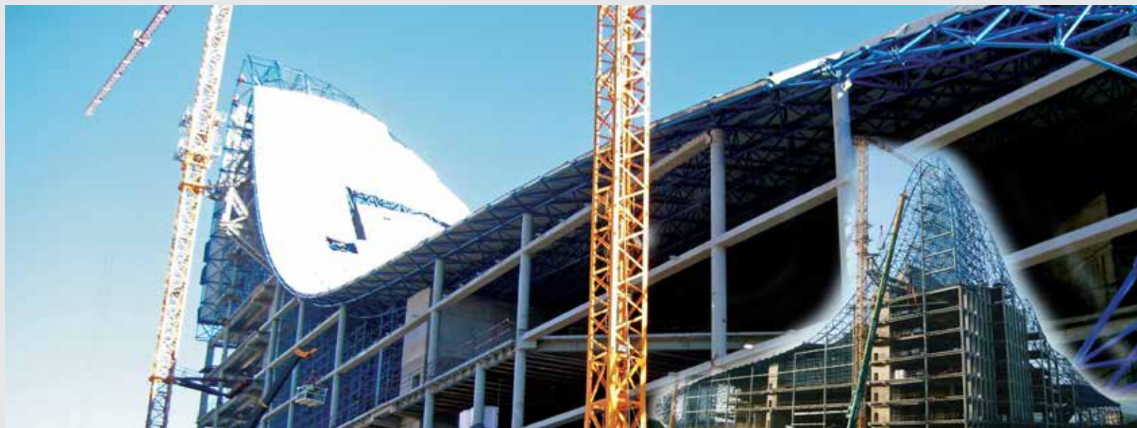
Haydar Aliyev Havaalanı, Dış Hatlar Terminali Çelik İmalat ve Montajı Bakü/AZERBAIJAN Haydar Aliyev Airport, International Terminal Steel Manufacturing and Erection Baku/AZERBAIJAN
