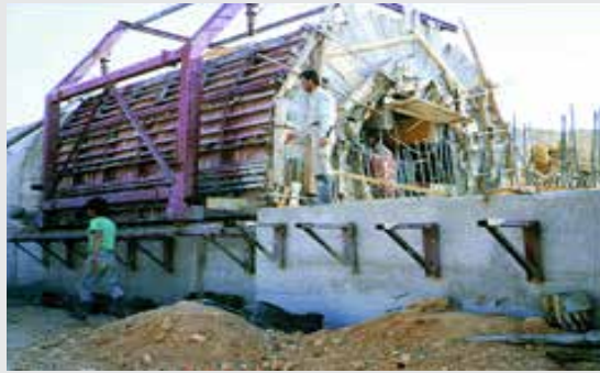
Deliçay Barajı Dipsavak Tüneli Karaman/TÜRKİYE Deliçay Dam Bottom Outlet Tunnel Karaman/TURKEY
