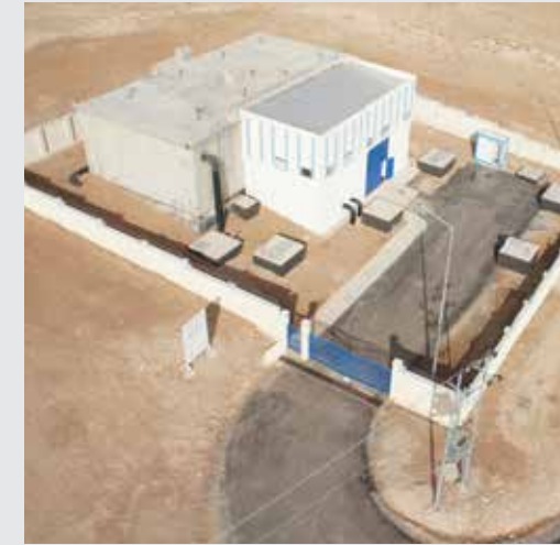
Domez Su Deposu / Domez Water Reservoir
