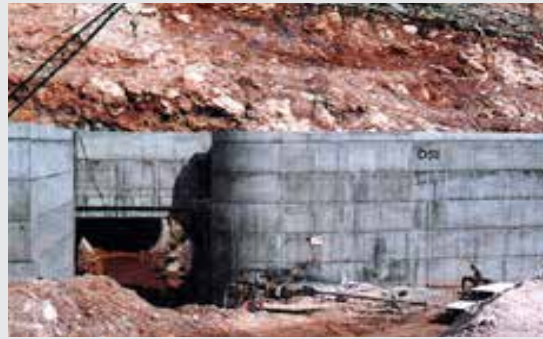
Akyar Barajı Dipsavak Tüneli Ankara/TÜRKİYE Akyar Dam Bottom Outlet Tunnel Ankara/TURKEY
